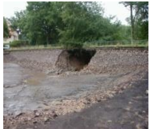
Exhibit 9: Erosion due flow of river and rain cuts (Erosion in Li Fyang Embankment in china)
