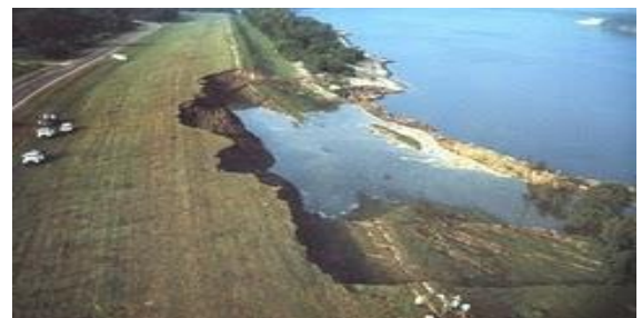
Exhibit 11: Erosion in Ukishwar Dam in Australia
