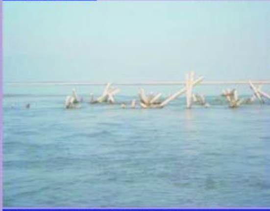
Porcupines used to tame the flow in kosi.
